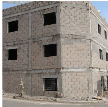
Fig. 8. Building of volcanic concrete blocks.
