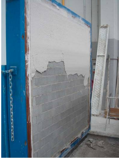
Fig. 10. Wall of concrete blocks with thermal mortar layer.
